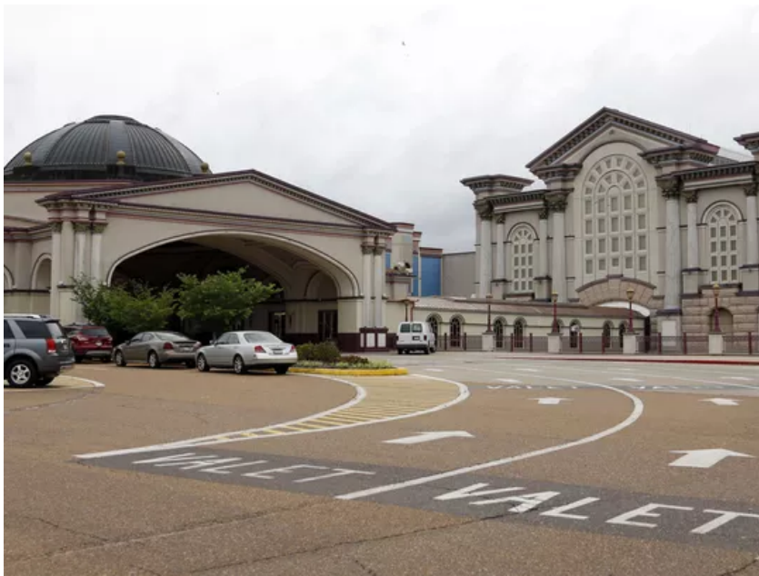
The former Harrah's Tunica casino is shown in this May 13, 2014, photograph. The casino closed June 2, 2014, and was demolished in Aug. 2015. The hotel buildings, convention center and golf course remain but are vacant. (Photo: Rogelio V. Solis, AP)
